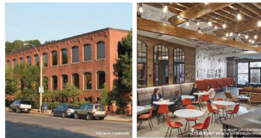
1210 Washington Street is a historic brick warehouse building that now houses the global headquarters of Rockport Shoes along with offices for VideoLink, a national leader in video production.
