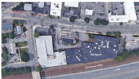
In 2017 Rockport Shoes moved its global headquarters to the historic brick warehouse in this block of West Newton Square.
